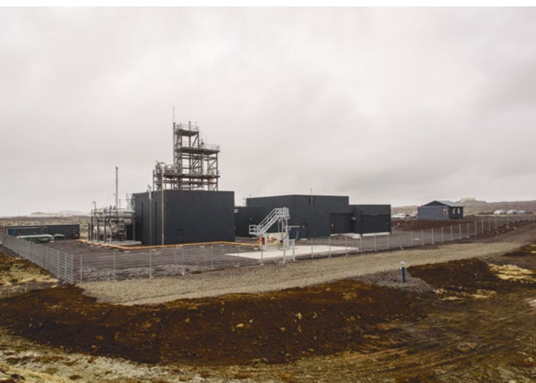
FIGURE 1 Carbon Recycling International – the world's first commercial power to CO 2 methanol plant, producing 4000 t of methanol and capturing 6000 t of CO 2 (© Carbon Recycling International)
